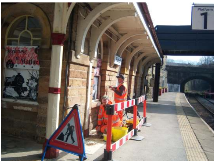
Stonemasons renovating Matlock Station
