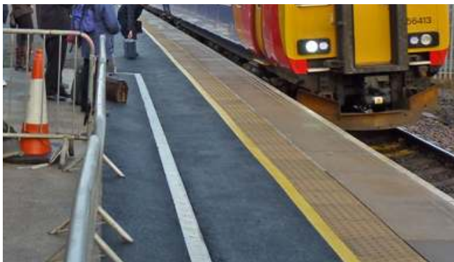
Duffield platform resurfaced
