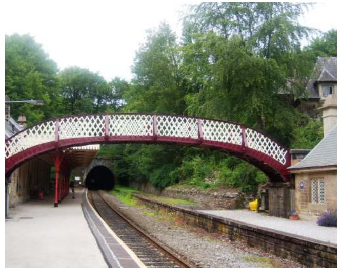
Cromford footbridge repainted in traditional Midland Railway colours
